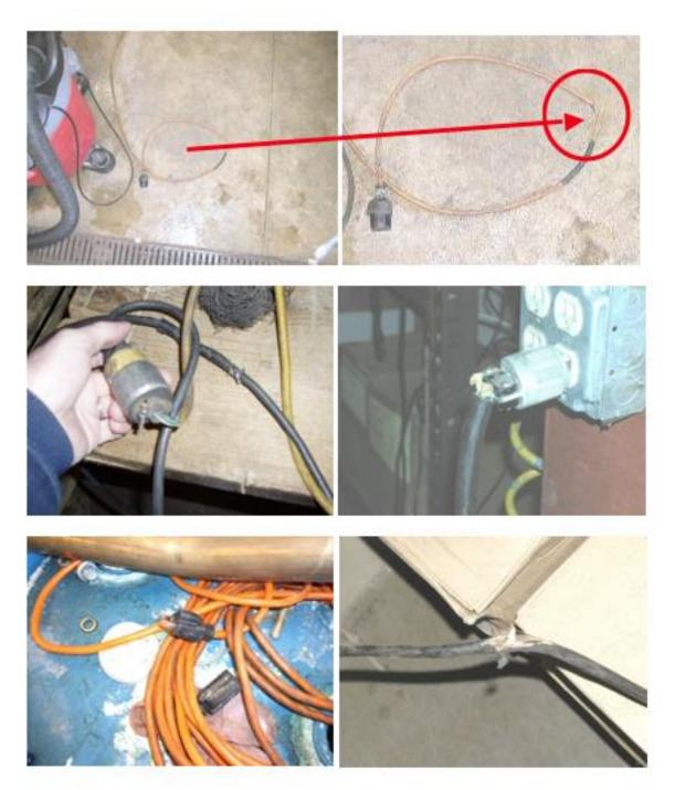
**Substitute for Fixed Wiring**: Flexible cords like extension cords cannot be used as a substitute for fixed wiring, or run through holes in walls, ceilings, or floors. They cannot be attached to building surfaces or concealed behind building walls, ceilings, or floors.
